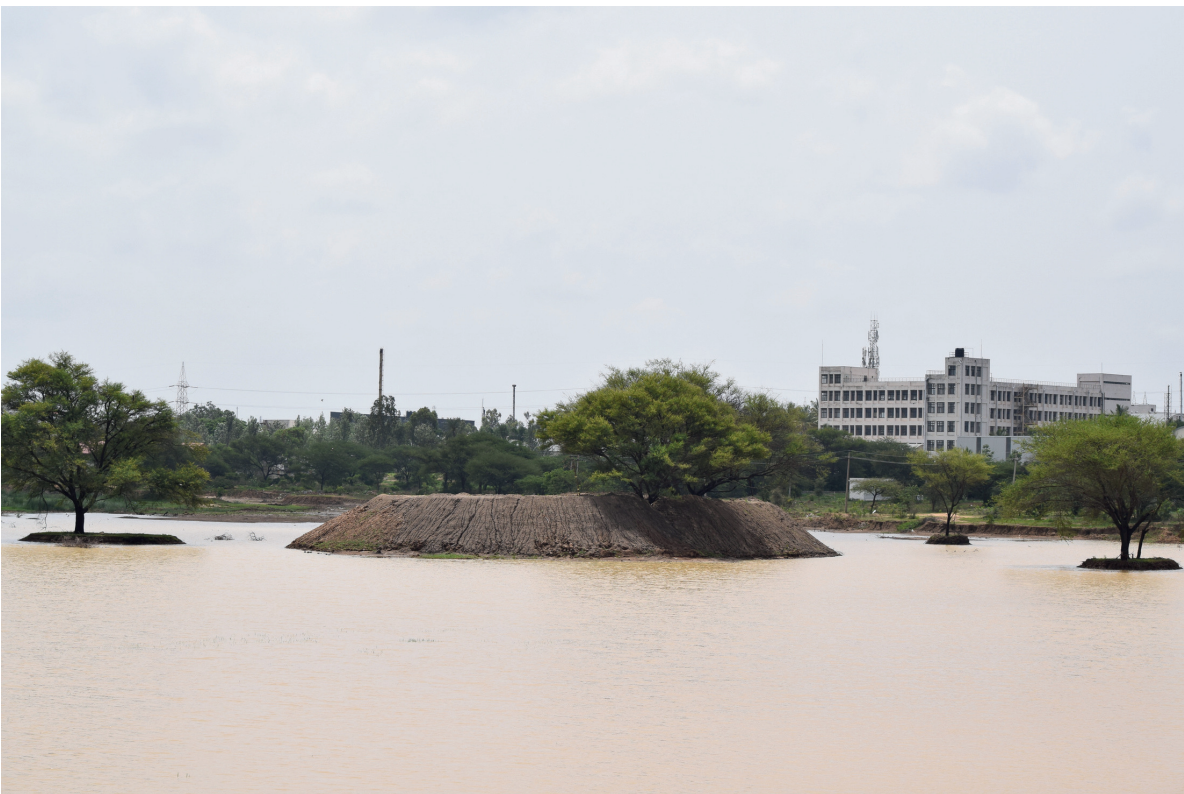
After Rejuvenation - June 2019
